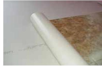
3. Install foam underlayment (Except Malibu and Worthington). When installing over concrete, install an approved vapor retarder prior to installing foam underlayment.
