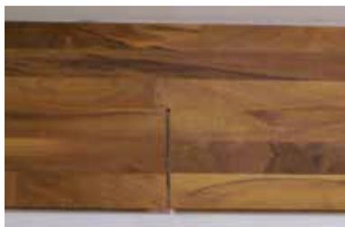
13. Slide plank toward previous plank. Position approximately 1/4" away from previous plank.
