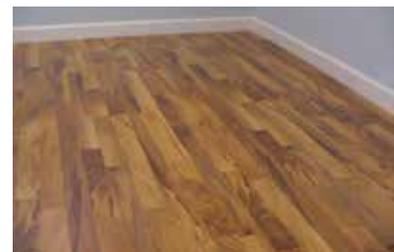
15. Continue until entire room is complete. Use of T-molding is required for rooms over 40'. Remove spacers and install matching quarter round and moldings.
