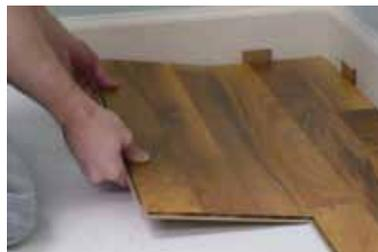
11. Install first plank of second row by inserting tongue side of plank at a low angle into groove side of previous row. Rotate plank downward until flat. Do not use tapping block to install long side of planks.
